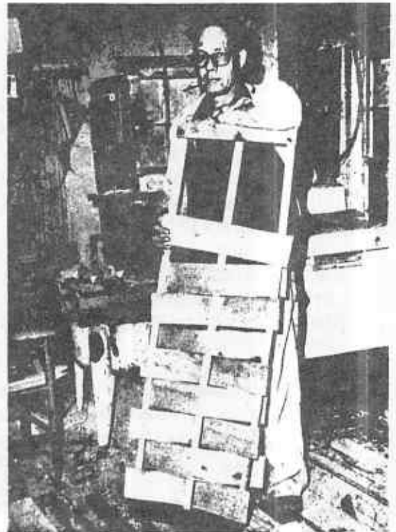
Jack McCutcheon. Ladder-back slats are placed in shaping rack for curing.
